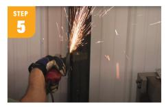
Be sure to grind off the mill scale on the base plates and vertical post to which the stand will be attached.
