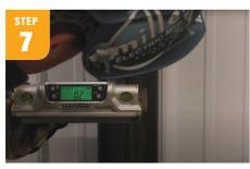
Grab your digital level and make sure your top base plate is level; check both directions before welding in place.
