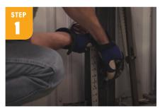
Measure where to place your top and bottom base plates to mount the equipment stand to the vertical post. The bottom swivel plate and mounting base will be attached by a diagonal support tube to help support the weight.
