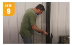
Before drilling your holes in the mounting base, check to make sure your clearance is at least 1" from the weld.
